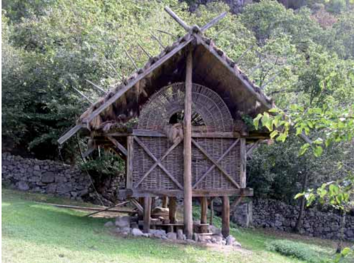
Plate 1. Jack's House (Photograph: J. Pilkington)
