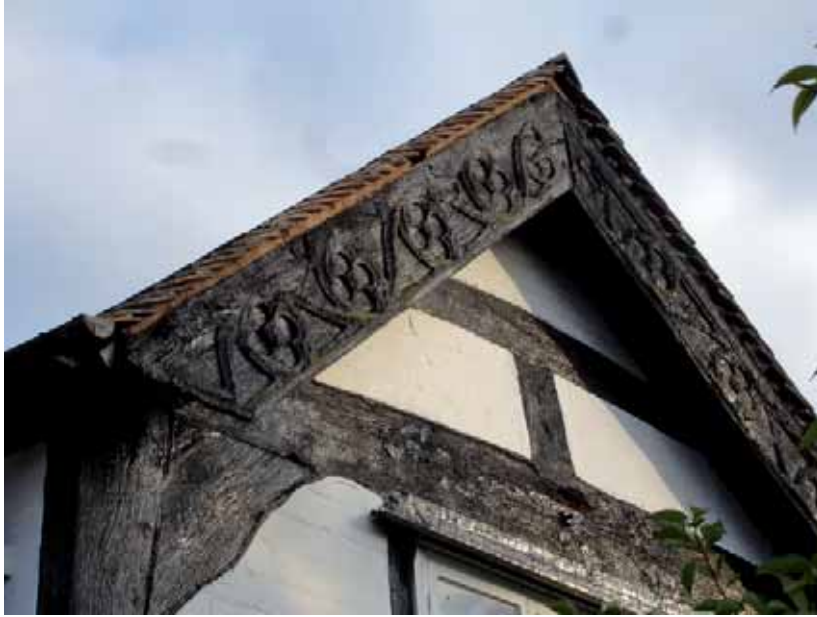
Plate 6. A carved medieval barge-board from a 15 th century status dwelling in Weobley, Herefordshire (Photograph: G.H. Nash)
